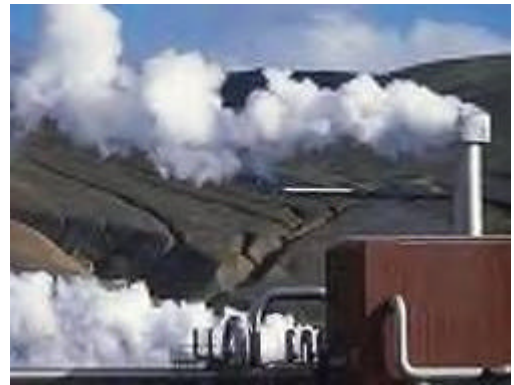
Geothermal energy plant
